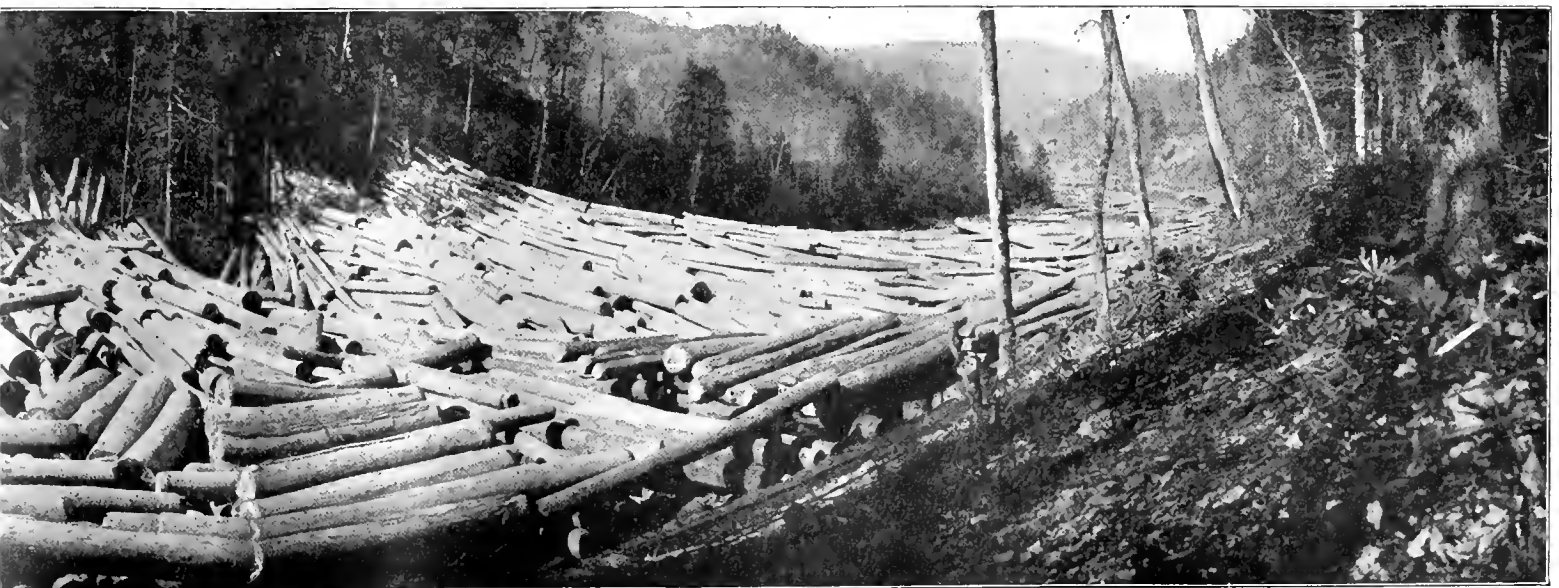
WITH THE AID OF A CONCRETE SPLASH DAM, 350 FEET IN LENGTH AND 25 FEET IN HEIGHT, LOCATED ONE-HALF MILE BELOW THIS LOG DUMP, THESE LOGS WERE DRIVEN THROUGH THE BREAKS OF BIG SANDY RIVER TO PIKEVILLE, KY., AND THERE RAFTED AND FLOATED DOWN TO THE OHIO RIVER AT CATLETTSBURG, KY.
